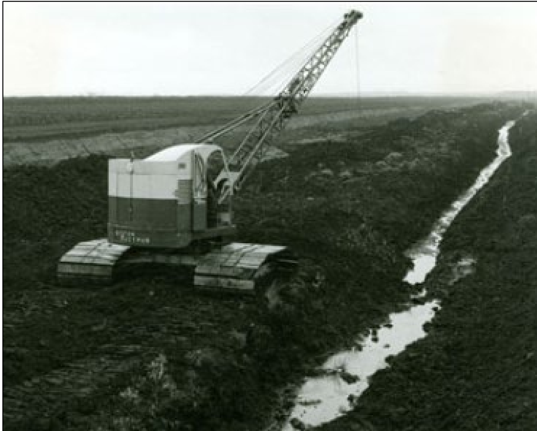
Plate 4-2: Dragline/Shovel Excavator (Source: https://www.bordnamonalivinghistory.ie/equipment-detail/draglineshovel-excavator/ )
