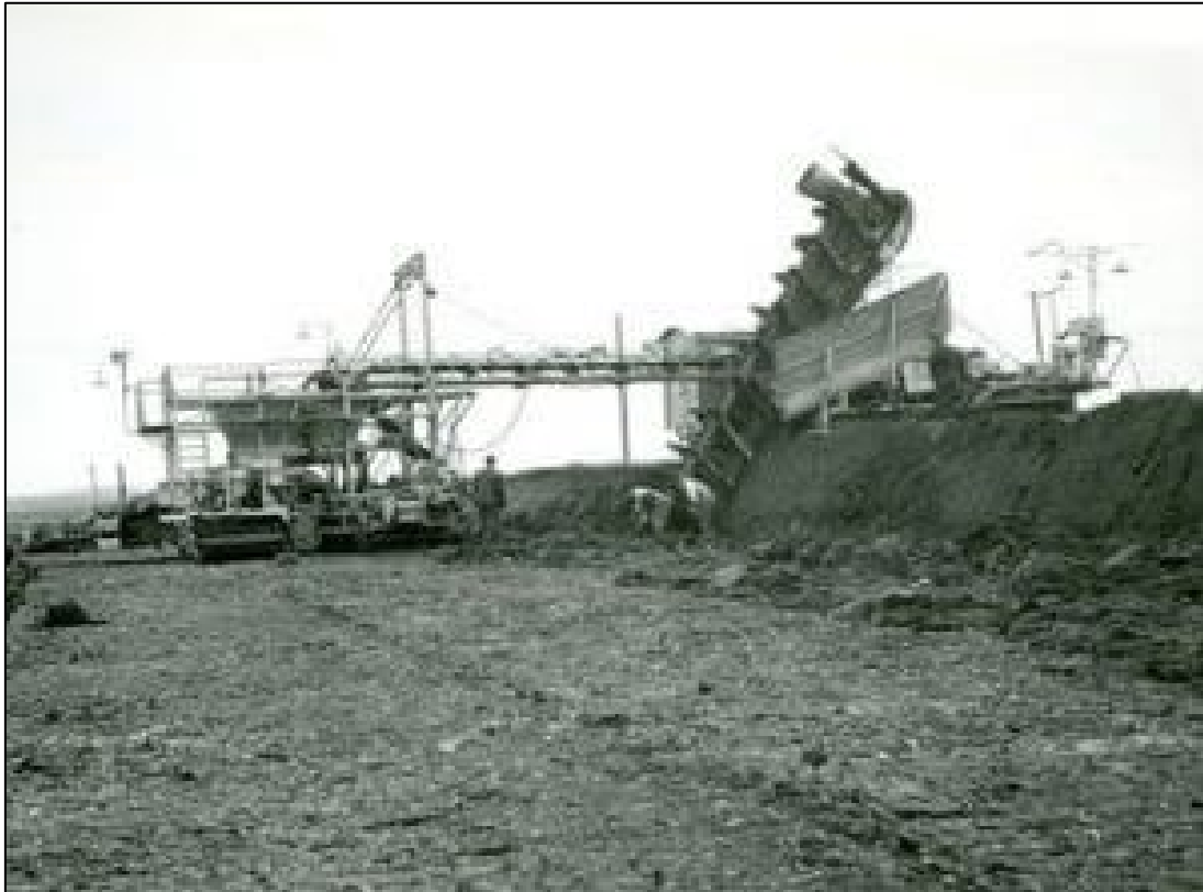
Plate 4-21: Sod Peat Bagger/Excavator. (Source: https://www.bordnamonalivinghistory.ie/equipment-detail/sod-peat-baggerexcavator/ )
