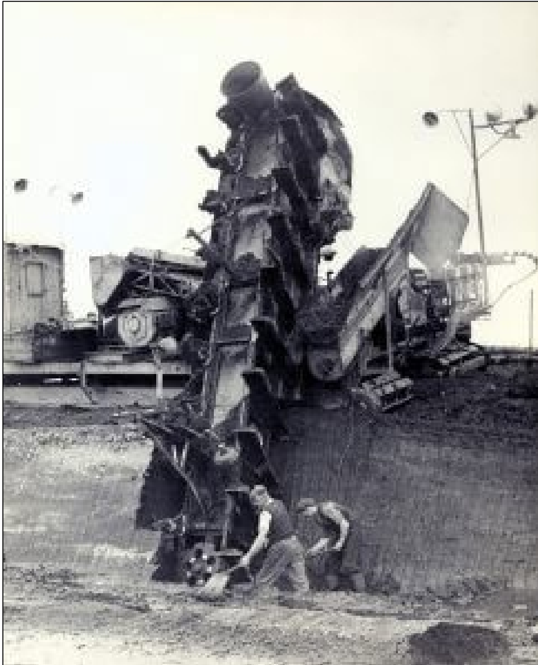
Plate 4-20: Sod Peat Bagger/Excavator. (Source: https://www.bordnamonalivinghistory.ie/equipment-detail/sod-peat-baggerexcavator/ )
