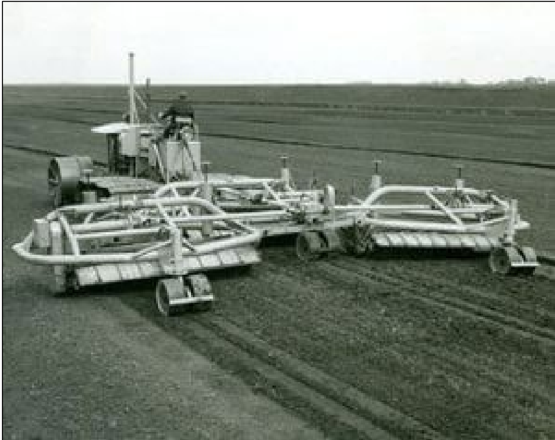
Plate 4-27: Triple miller attachment. (Source: https://www.bordnamonalivinghistory.ie/equipment-detail/miller-attachment/ )
