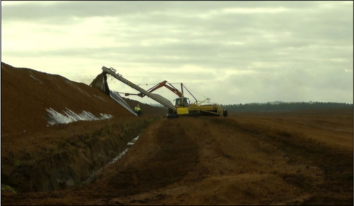
Plate 4-14: Polythene covering of stockpiles
